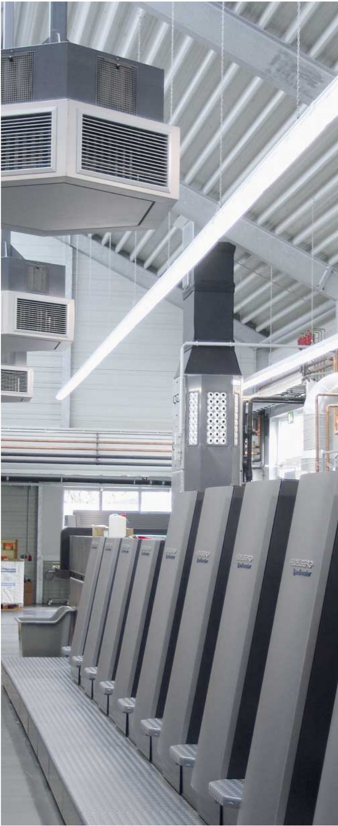
The new pressroom in Eltville. The Speedmaster CD 74 with air supply column in the background and Temcoil ambient air coolers on the ceiling.
