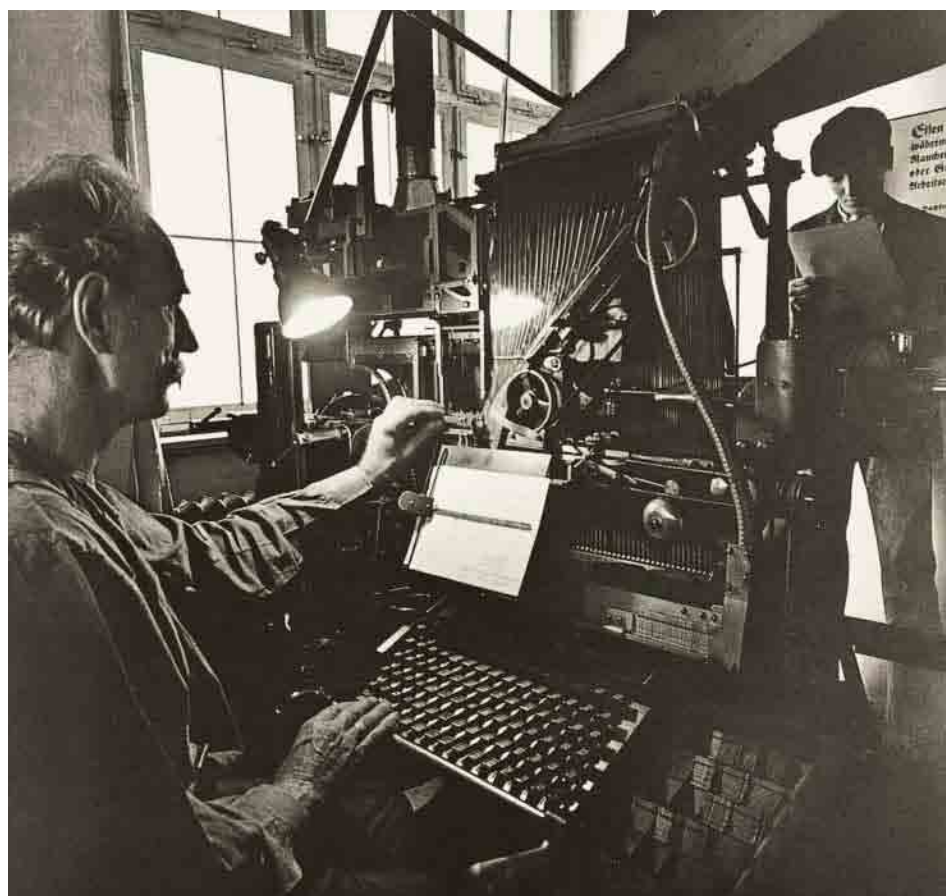
For decades, the "Linotype" dominated mechanical composition around the world. But after 1935, machines could be fed with punched tape. Linotype delivered its last lead composition typesetting machine in mid-1976.
